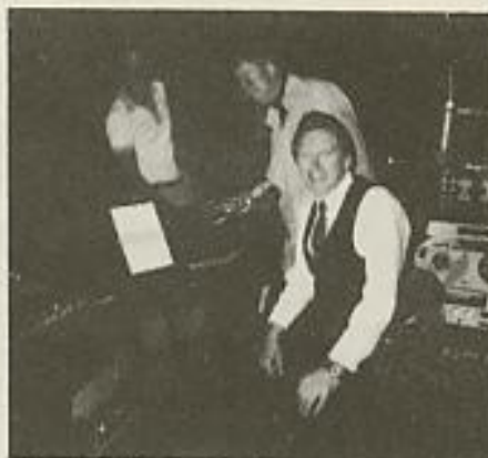
David Kantor, David Gray and Vern Grimsley inspect the newly-installed electronics in the audio control room.
